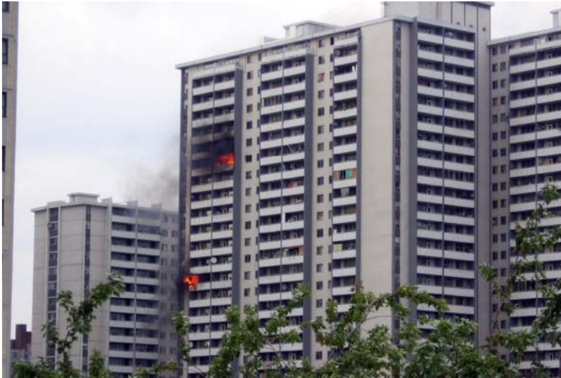
200 Wellesley Street – Fire (August 2010)
